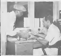
TOOL SLIPS for all shift transactions, above, are filed according to tool description and the craft making the request. Mr. Pantophlet checks off pneumatic tools with E. Richardson, below right.
